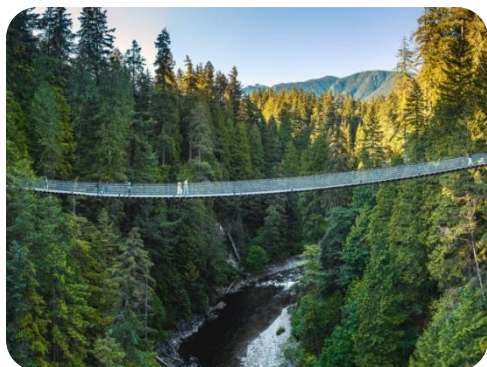
CAPILANO SUSPENSION BRIDGE
