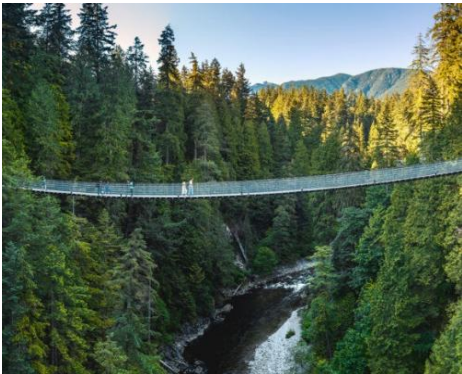
CAPILANO SUSPENSION BRIDGE
